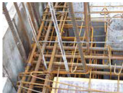
The end joint on the standard floor
