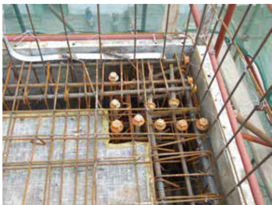
The end joint on top floor corner column
