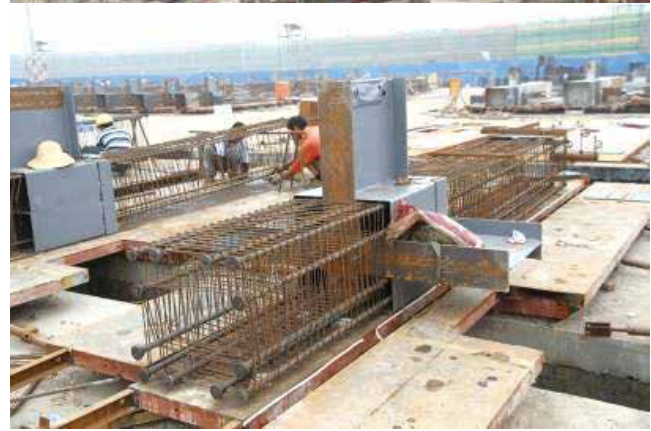
Precast concrete columns, Steel beams, Cast-in-place Slab Structure
