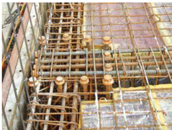
The end joint on top floor side column
